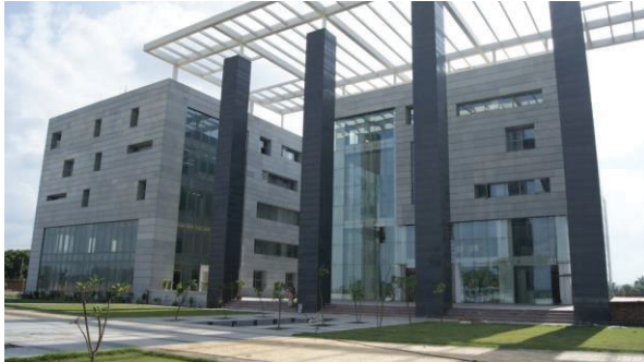
Academic Building Façade / Entrance
